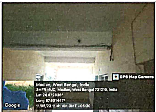
CC Camera 3 at Staff Room Corridor
